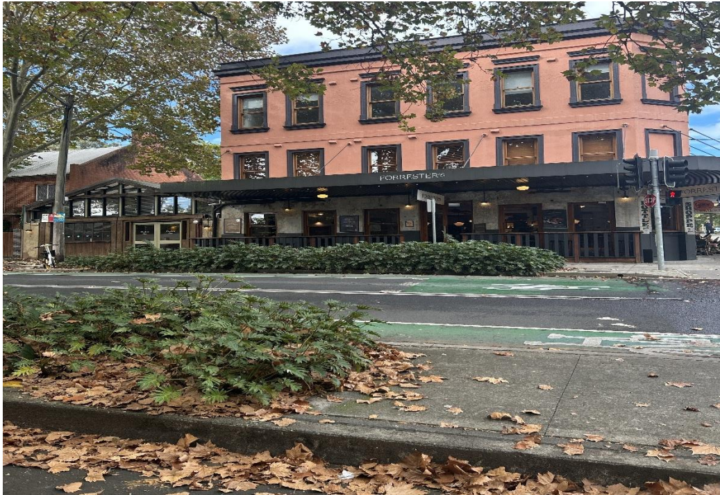
Figure 1: 332-338 Riley Street, Surry Hills, viewed from the west
